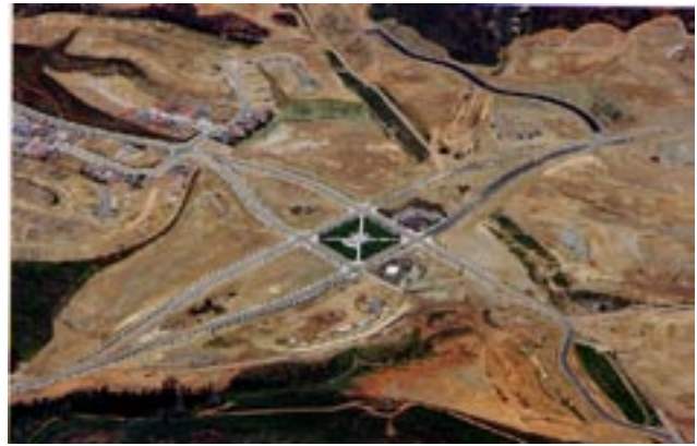
Illustration 5: San Elijo Village street couplet construction
